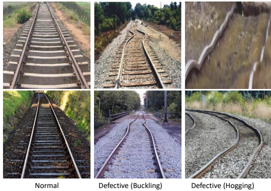
Fig. 4. Sample images from our Track Misalignment Detection (TMD) dataset.
