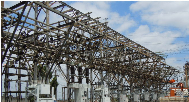
Fig. 2. Disconnect switches in a substation, among other structures and equipment. At least 27 switches are visible in this image.
