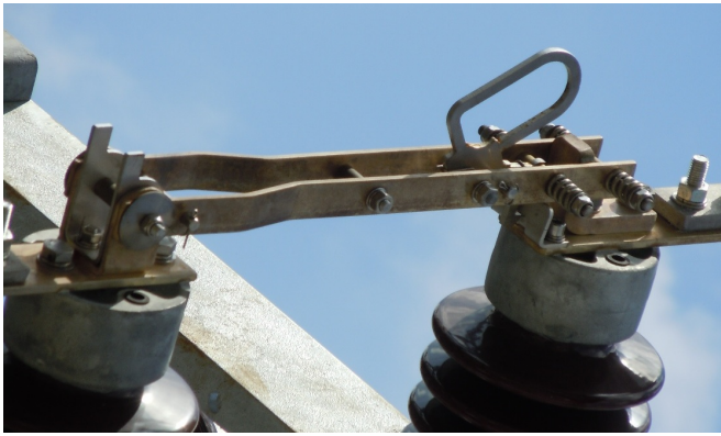
Fig. 1. Close view from a closed disconnect switch.
