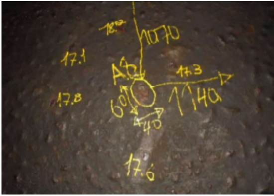
Fig. 1. Sample image of an FPSO tank with markings of previous inspections.
