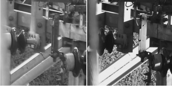
Fig. 10. Two captures of the same switch at different times. Although the state remained the same, differences in lighting make the conductive part darker than the background in the first capture, but brighter at some points in the second capture.
