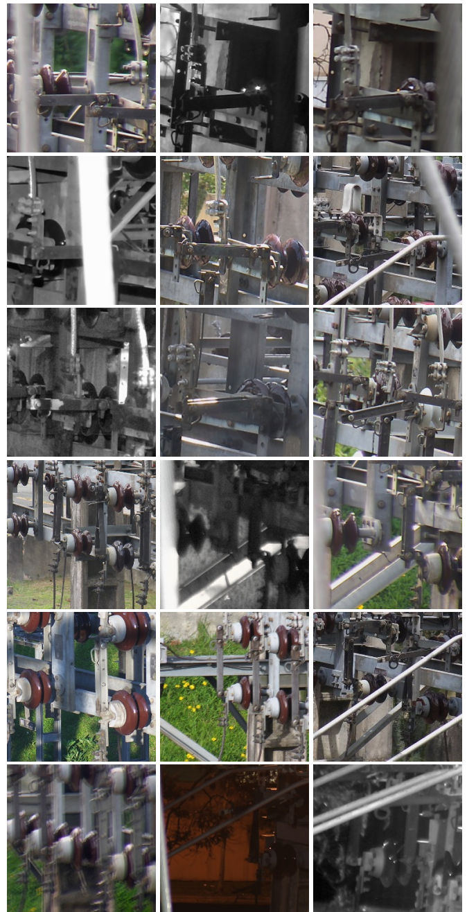
Fig. 3. Disconnect switches. All these switches have the same function and electrical specification. Each image shows a switch with its base point at the lower right quadrant. In the uppermost 9 images, that switch is open, in the bottommost 9 images, it is closed.
